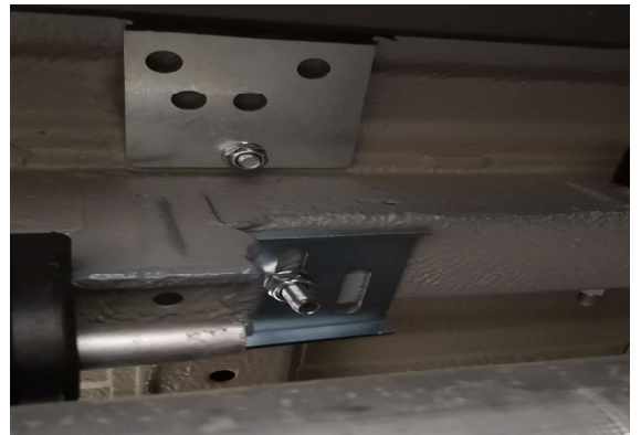
Reinforcements mounted on the right side.
