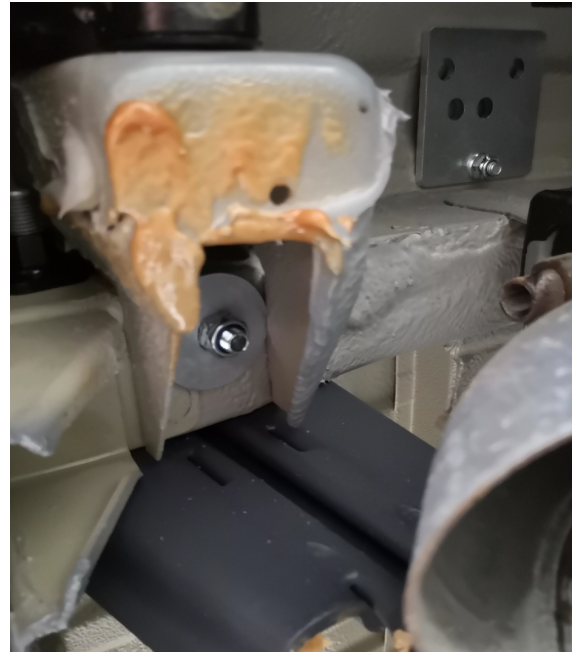
Reinforcements mounted on the right side.
