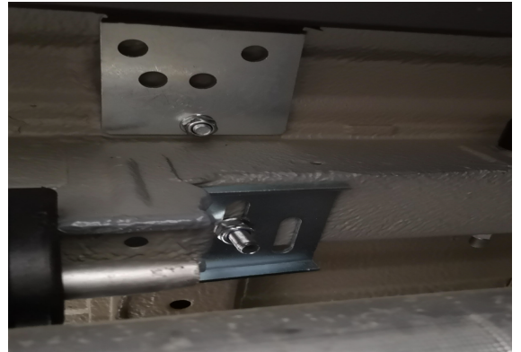
Reinforcements mounted on the right side.
