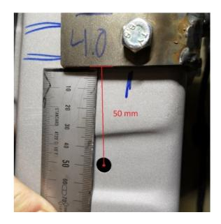
Keep a distance to the marked hole of 50 mm.
